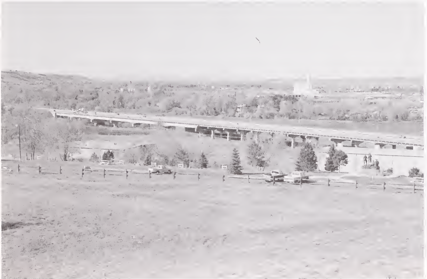
At the time of its construction in 1951, the O. S. Warden Bridge in Great Falls was the longest bridge in Montana (it was surpassed by the new Yellowstone River Bridge in Billings in 1992). Built by the Anderson Construction Company, the Warden Bridge consists of 21 approach spans and six main spans.
